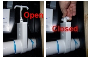
Figure 15 - Valve Open/Closed
